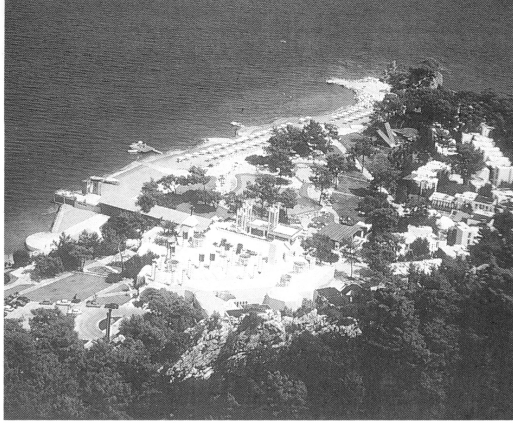
(e) Aerial view of site
